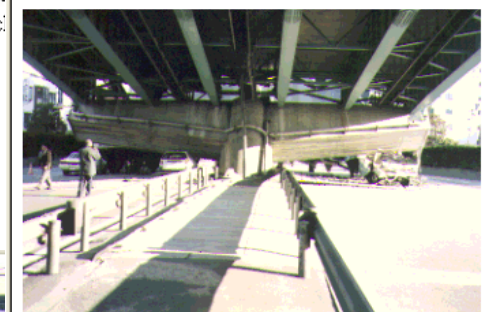
Photograph A2 Hanshin Expressway Bridge in Nishinomiya City. The photograph, taken under the collapsed deck, shows that the reinforced concrete pier is leaning sideways.
