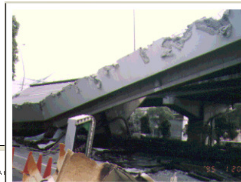
Photograph I3 Route 43 Iwaya Viaduct collapsed. Viewed from the north, the deck is leaning to the north.
