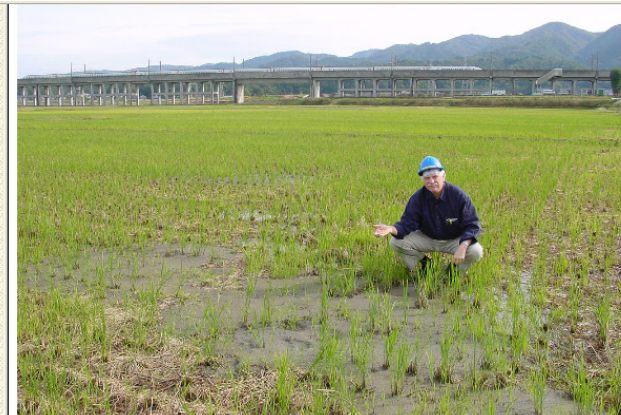
Figure 14. One of the possible explanations proposed for the Shinkansen derailment was the large amplitude of the transient viaduct displacement induced by the softening of the liquefied ground (10/31/2004 10:04:42 AM, N37.39094 E138.84270).
