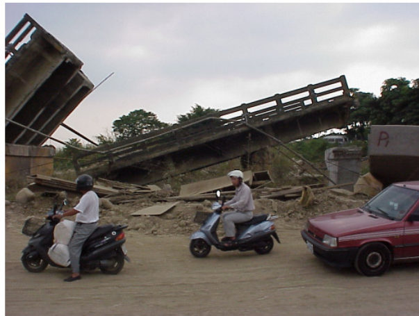
12. Collapsed bridge spans near Highway 129/136 intersection near Taiping (N 24.1335 E120.7352). The longitudinal direction for the bridge has an azimuth of approximately 300 degrees. The fault is known to pass beneath the bridge based on exposures west and east of the spans, but its precise location is unknown due to grading near the bridge. View in photo is to the NE. Note the spans have been pushed to the SE (to the right in the photograph) off their supports, possibly from compression associated with the faulting.
