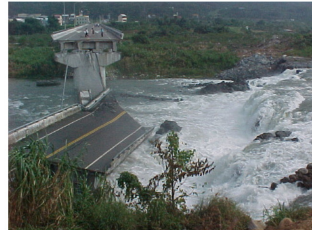
1. Waterfall created by reverse fault movement just north of the south abutment of heavily damaged multi-span bridge north of City of Fengyuan and to the west of the Shihkang Dam (N 24.2786 E 120.7592; 9/30/99)
