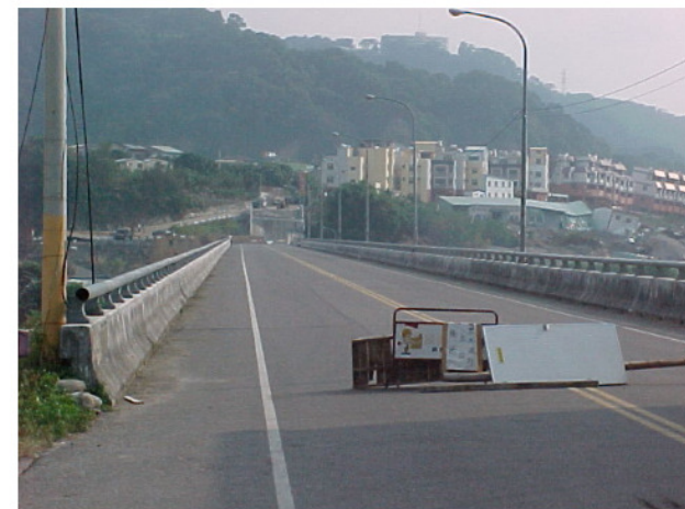
2. View to south showing right lateral offset of about 3 to 4 m and uplift or about 4 to 5 m in this bridge (N 24.28 E 120.76; 9/30/99)
