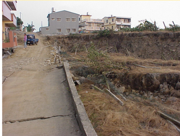
11. Close-up view of headscarp above collapsed bridge (N24.2854 E120.7969).
